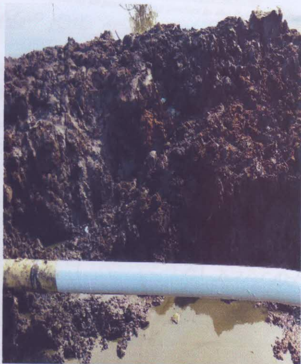
LEAK POINT AFTER REPAIR
